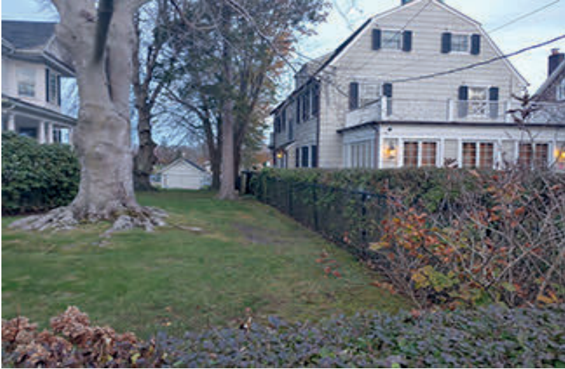
Fig. 3 Photo showing the north (rear) and west sides of the horror house and its distance from the neighbor on the north side. The narrow projection from the north wall is the rear entrance to the house.
